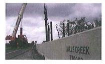
RiverWalk Extension Pedestrian Bridge Pictured are the H-Piles being driven at Mills Creek for the pedestrian bridge that will be part of the new RiverWalk extension on Seminole Boulevard. The four iron pilings were driven with a pneumatic hammer to a depth of 80 feet and will support the concrete foundation that the bridge will be attached to.
